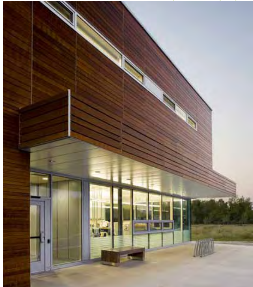
The Sûreté du Québec headquarters building For Laval, Laurentides and Lanaudière is certified BOMA BEST Level 4 and LEED Gold.
